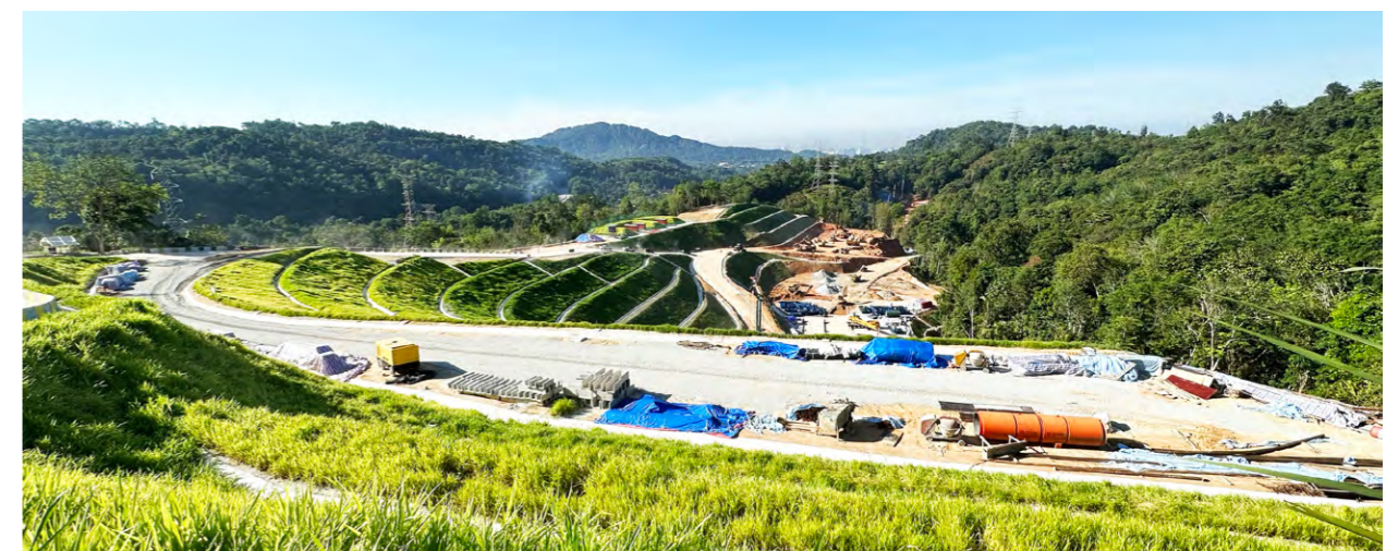
► Water and soil conservation measures in tunnel construction
