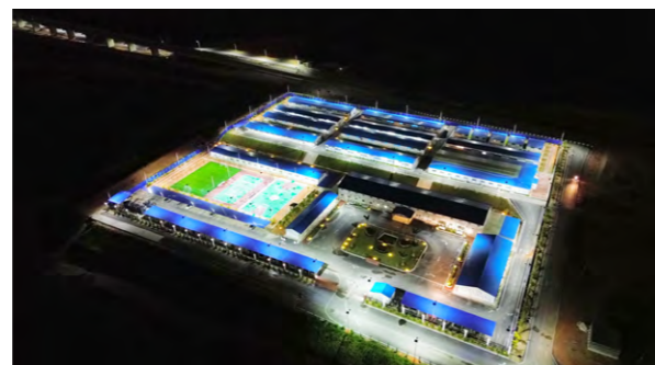
► Road lighting project adopts solar clean energy
